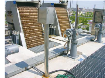
齿耙格栅 Rake Bar Screen
