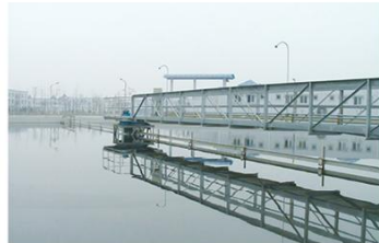
BZBG半桥式周边传动刮泥机 Half Bridge Peripheral Drive Sludge Scraper
