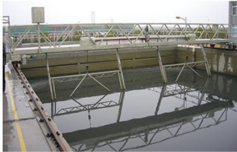
桁架刮泥机 Bridge Sludge Scraper
